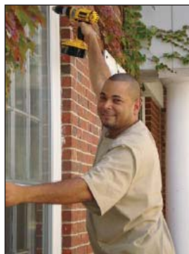
Luis Martinez, Director of Maintenance prepares for the new windows
